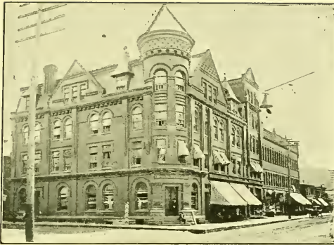
The Blennerhassett Hotel Building on Market Street.
